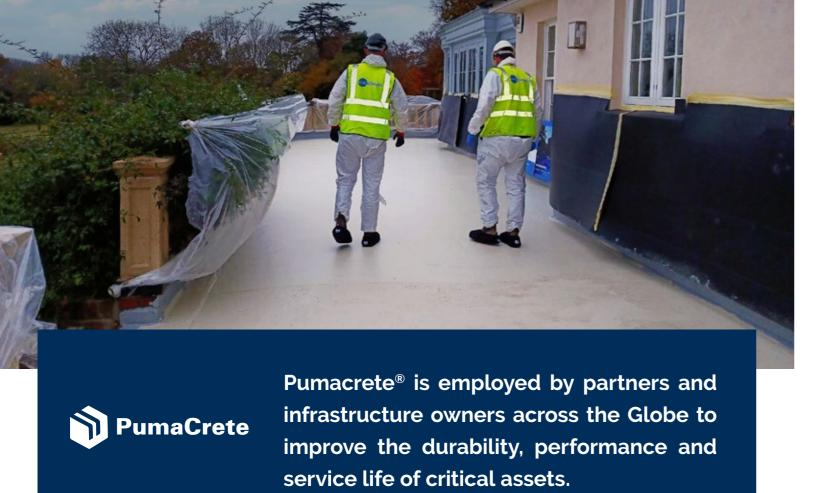
Formulated for application like an MMA with cured performance superior to a high grade Polyurethane. This unique chemistry prevents the degradation of deck surfaces on new structures and restoration projects.
