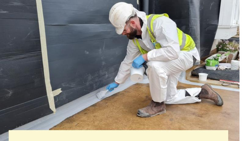
Pumacrete<sup>®</sup> is a two-part liquid applied polymer membrane system, based on Urethane-modified Acrylic Monomers (PUMA technology), and is used as a waterproof membrane for concrete structures, and for internally and externally applied tanking below and above ground.
